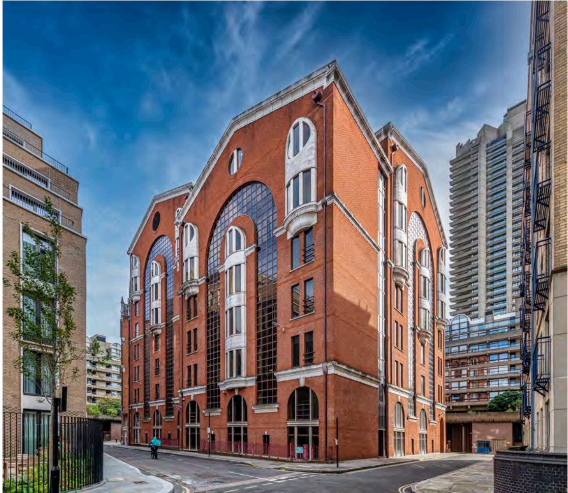
Image 2: View of rear of existing building from north-west – corner of Brackley Street and Viscount Street
