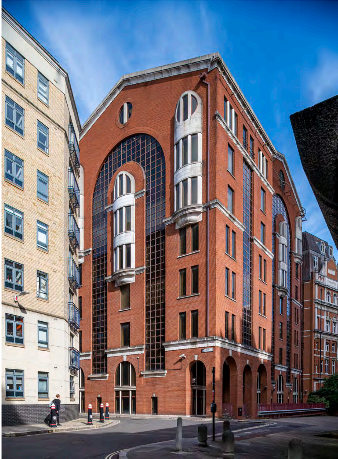
Image 3: View of existing building from south-west – taken from Bridgehouse Street showing corner of Viscount Street and Cripplegate Street
